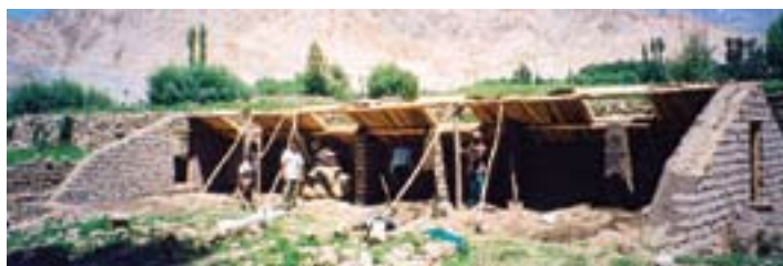
Picture 2: a greenhouse under construction (notice: roof, double walls, ventilation openings, angles)
