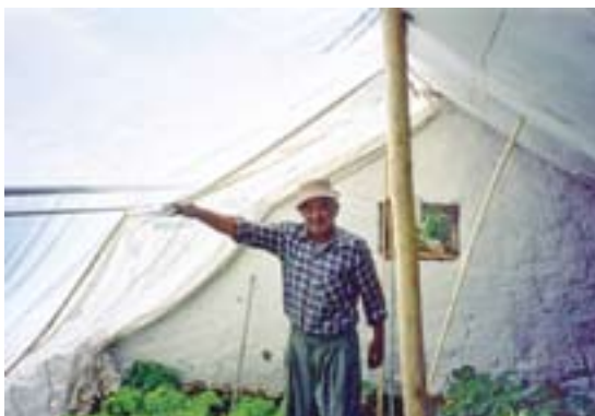
Picture 5: Inside view of a greenhouse (notice: curtain installed for night insulation, ventilation system)
