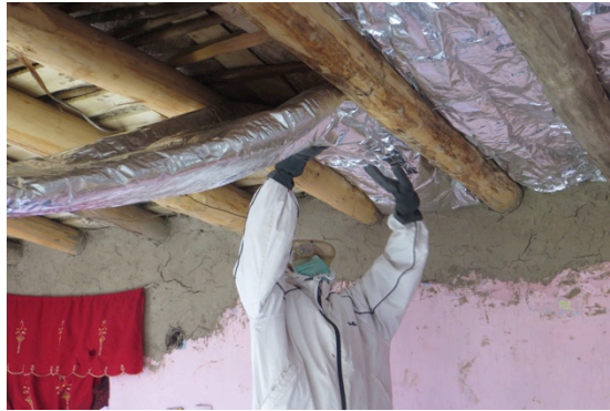
Fitting Roof Insulation
