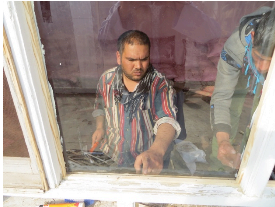
Fitting Double-Glazing
