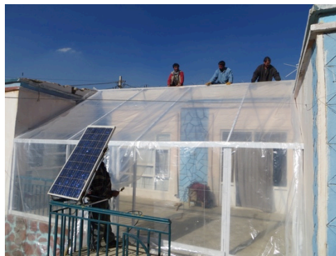
Covering a metal framed veranda with plastic coverings
