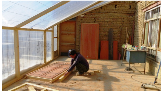
Making a wooden framed veranda with plastic covering
